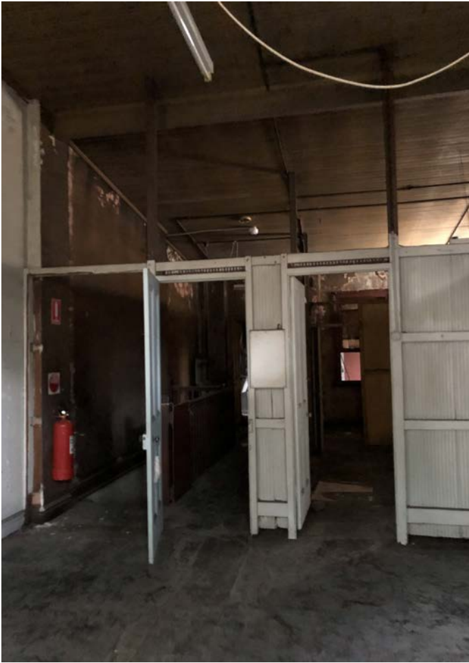
Figure 9: Second floor partitions, 84 Dixon Street.
