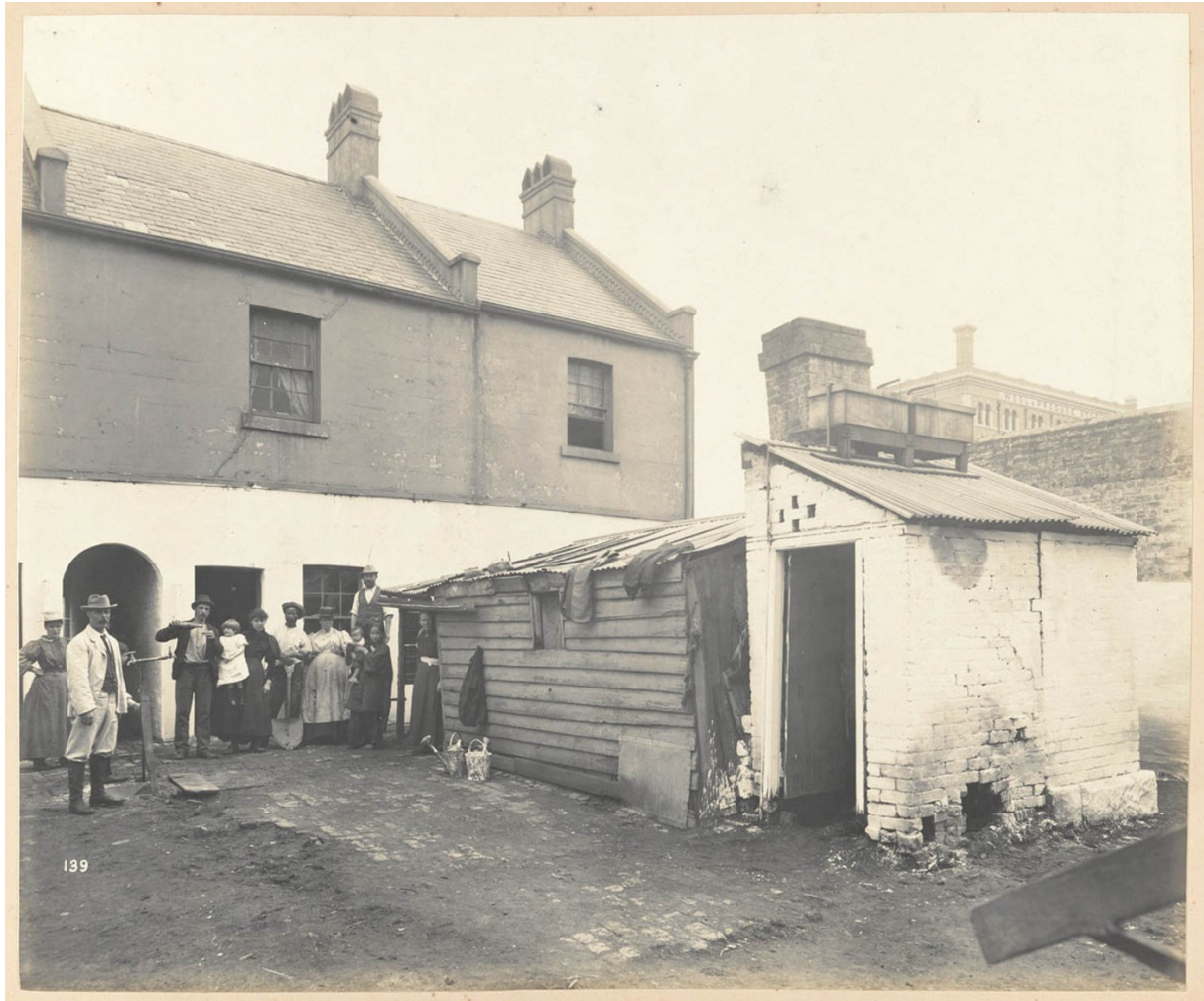
Figure 1: 'Rear of 84, 86 Dixon Street', 1900. These buildings were demolished prior to the construction of the current buildings in the early 20 th century. (Source: Views taken during Cleansing Operations, Quarantine Area, Sydney, 1900, Vol. III / under the supervision of Mr George McCredie, F.I.A., N.S.W. ff 138-9 (State Library of NSW)).
