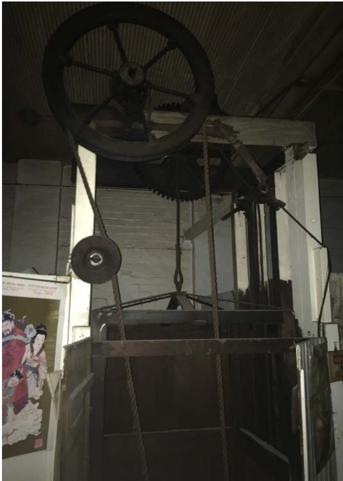
Figure 4: Goods lift mechanism.
