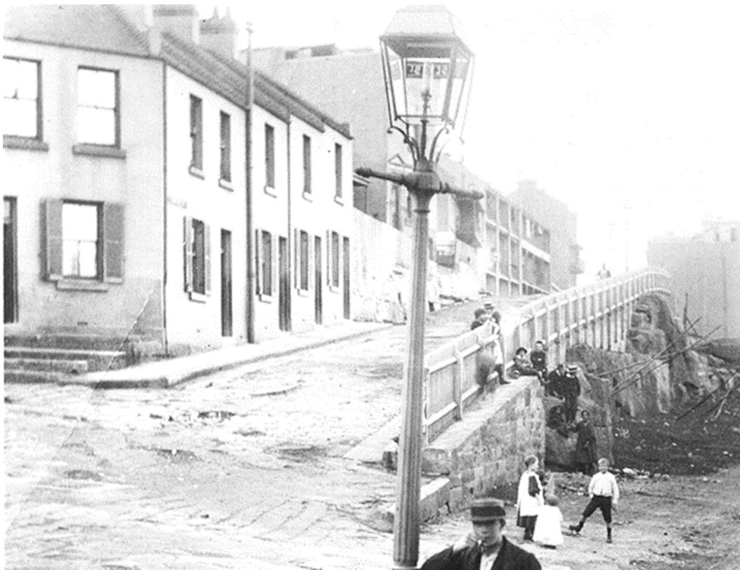
Figure 22 1901 configuration of Harrington Street, viewed from the corner of Essex Street. Note retaining wall along Harrington Street.
