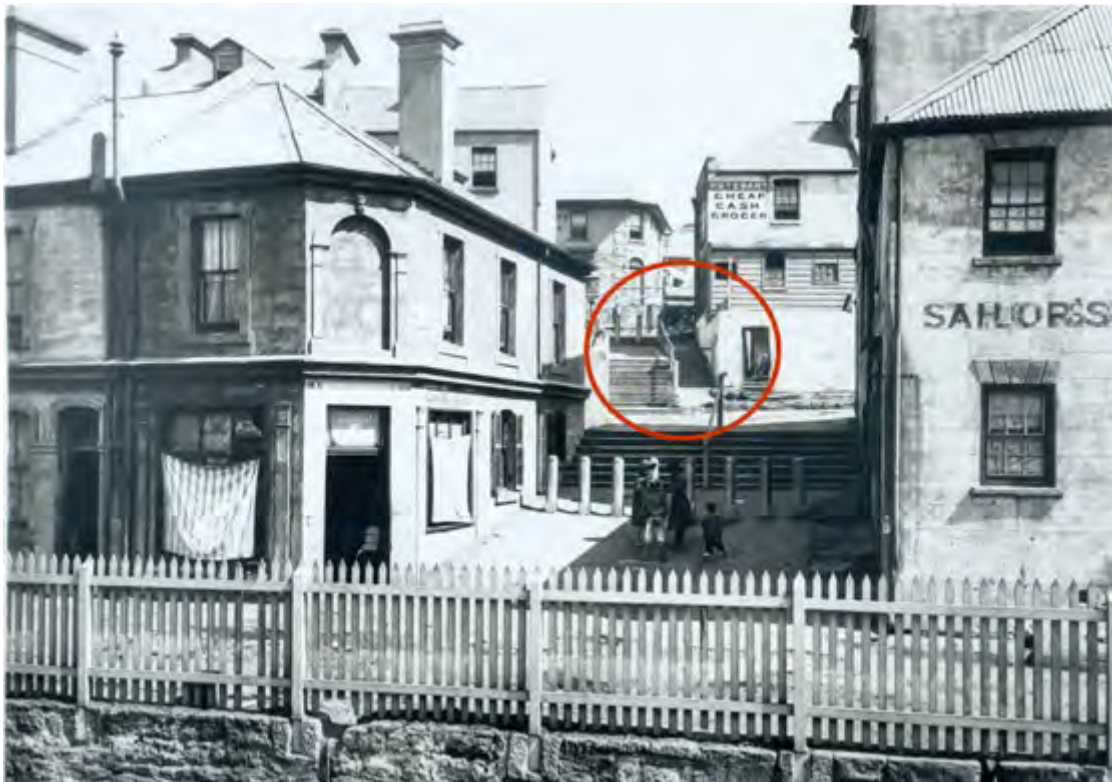
Figure 27 1901, Cumberland Place from Harrington Street. Note that there were no direct stairs from Harrington Street. Harrington Street was divided into two levels and a staircase was located south of Cumberland Place (to the left of the frame). The two steps to Cumberland Street (in the distance) were not shown in historic plans, including those created around this date. Note the goat protruding its head from the rear of yard of Susannah Place (circled) and posts fitted to prevent carts from going down the steps.
