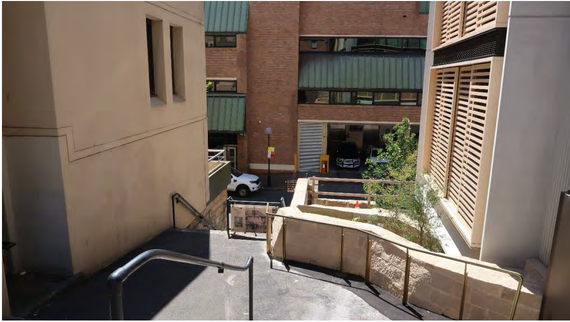
Figure 70 New sandstone wall and landscaping to 85 Harrington Street
