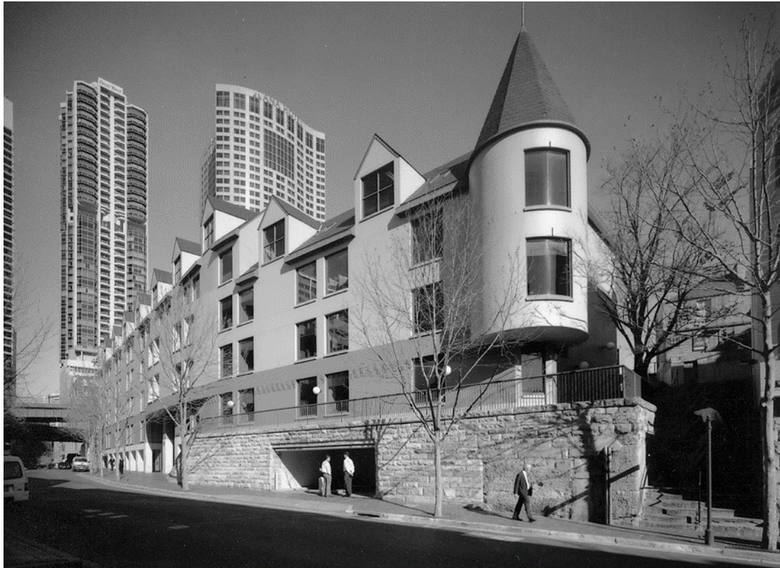
Figure 35 Harrington Street, 2001, QBE Office Building. Compare Figure 33, Figure 36 and Figure 27. Note Separation in the stairs.
