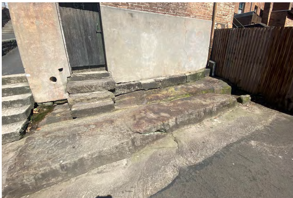
Figure 69 Rocky Sandstone outcrop at the rear of Susannah Place, Cambridge Street.
