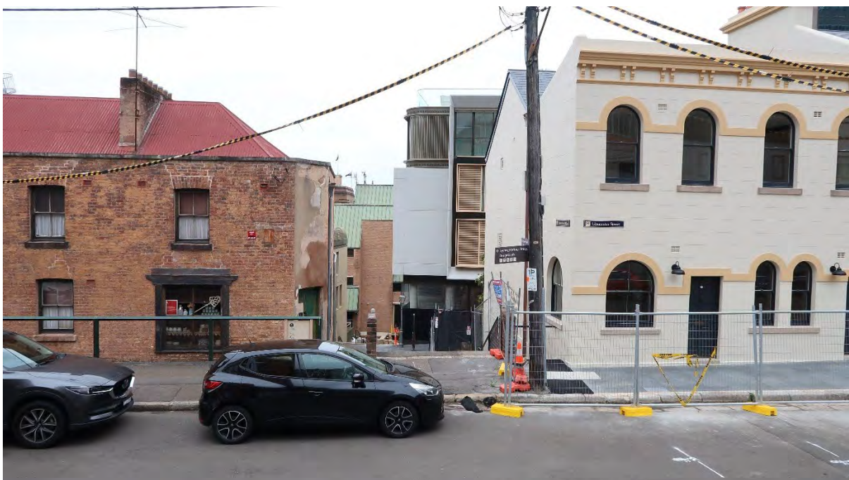
Figure 65 View through Cumberland Place and Steps to Harrington Street. Susannah place is to the left of the image and Bakers Terrace to the right.
