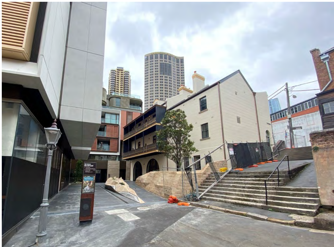
Figure 71 New wall at the rear of Bakers Terrace, now forming the boundary to Cumberland Place and Steps and replica gas lamp.
